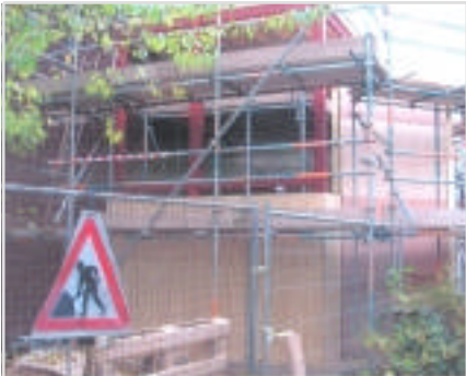
Renovating St Mathews's buildings
